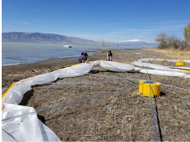
Figure 7 Limnocorral construction on the shore of Utah Lake.
