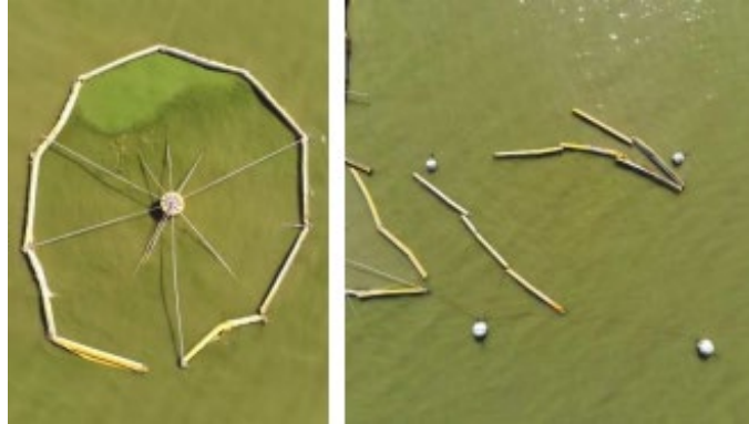
Figure 10 Corral structural damage after high winds and waves in Utah Lake.
