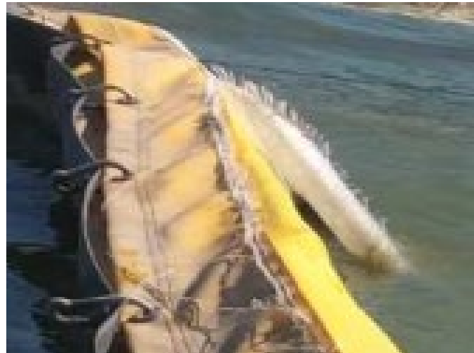
Figure 11 Corral damage after high winds and waves in Utah Lake.
