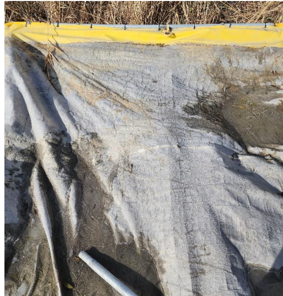
Figure 3 Corral #1 Wear and Tear
