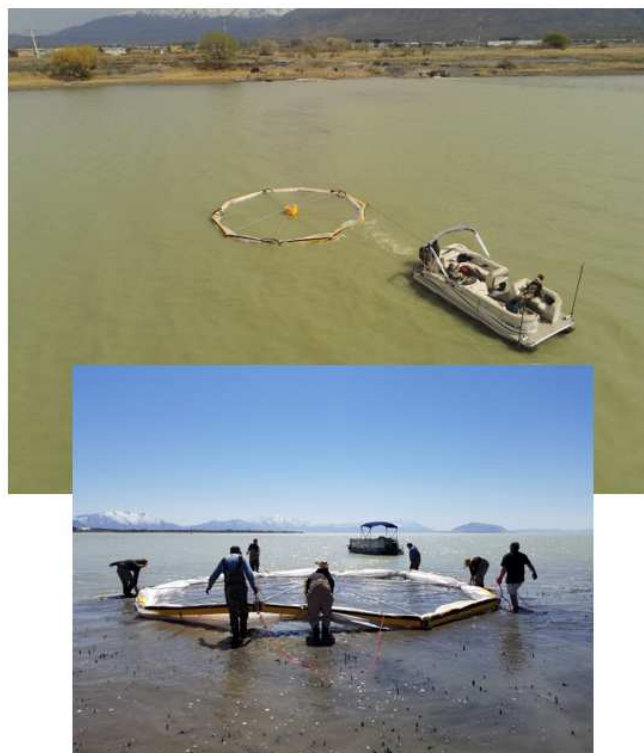
Figure 3 Limnocorral Installation
