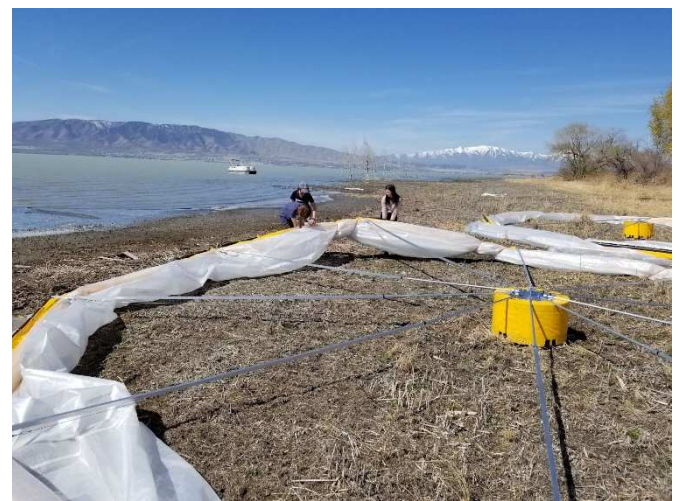
Figure 1 Limnocorral Construction
